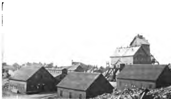
A. TAMARACK MINE.
